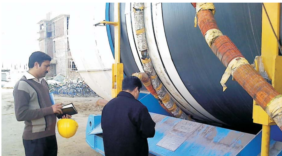
PNRA Engineers Inspecting Reactor Pressure Vessel of C-2
