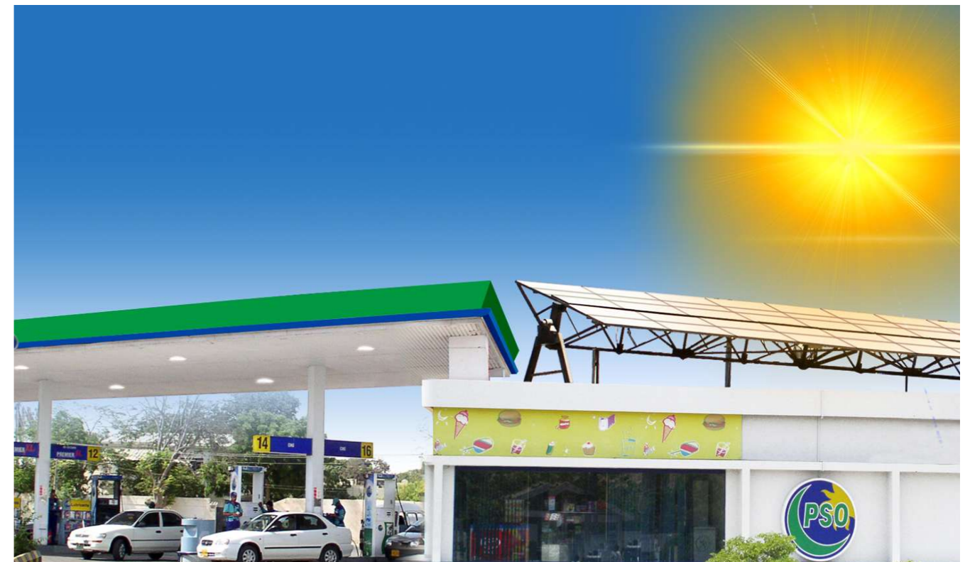
Solar Power at PSO Station
