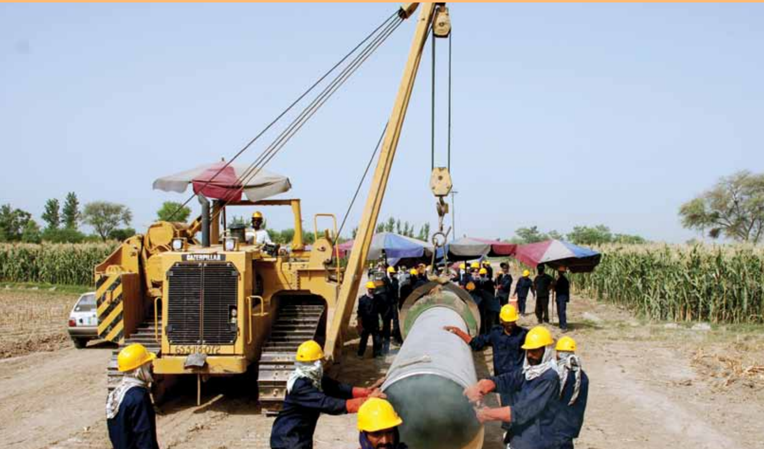
Work in progress of 36" dia Multan-Sabiwal line
