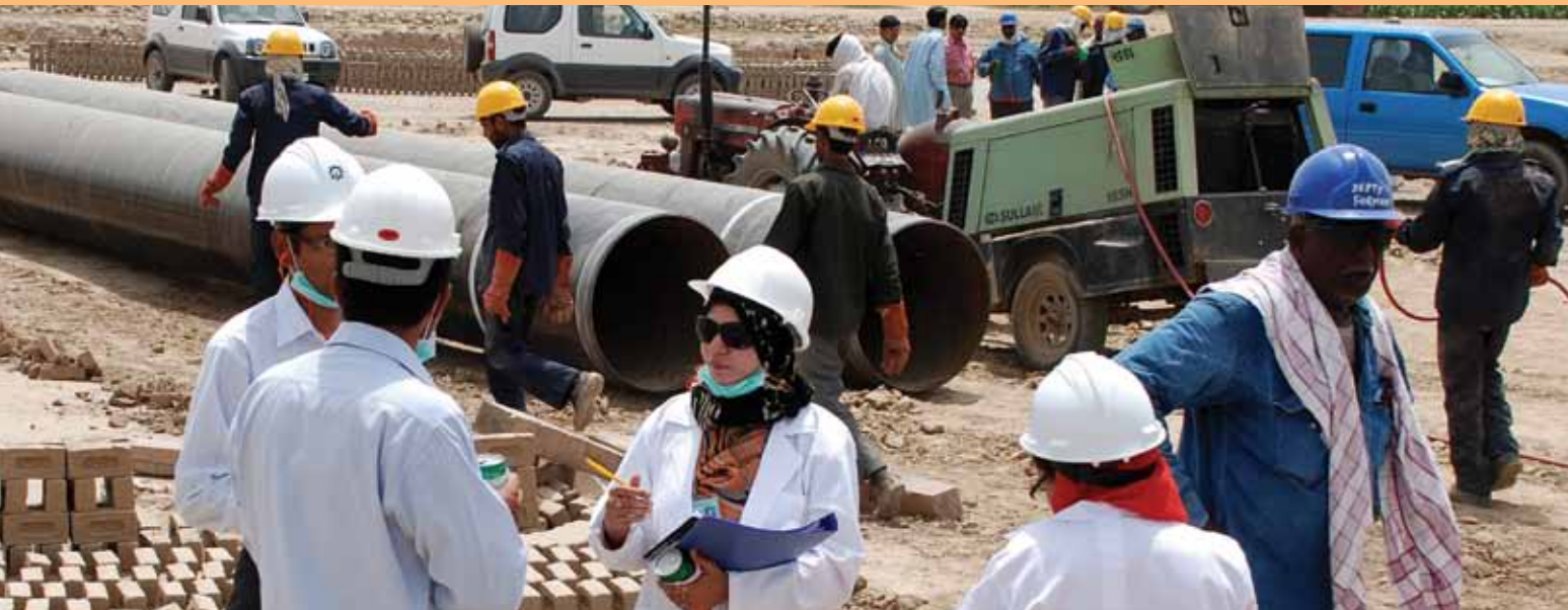
HSE team visit at 36" dia Multan-Sabiwal line
