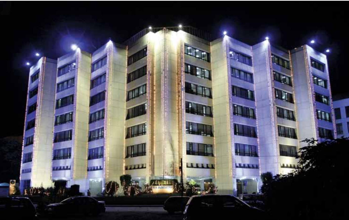
SNGPL - Head Office Building.
