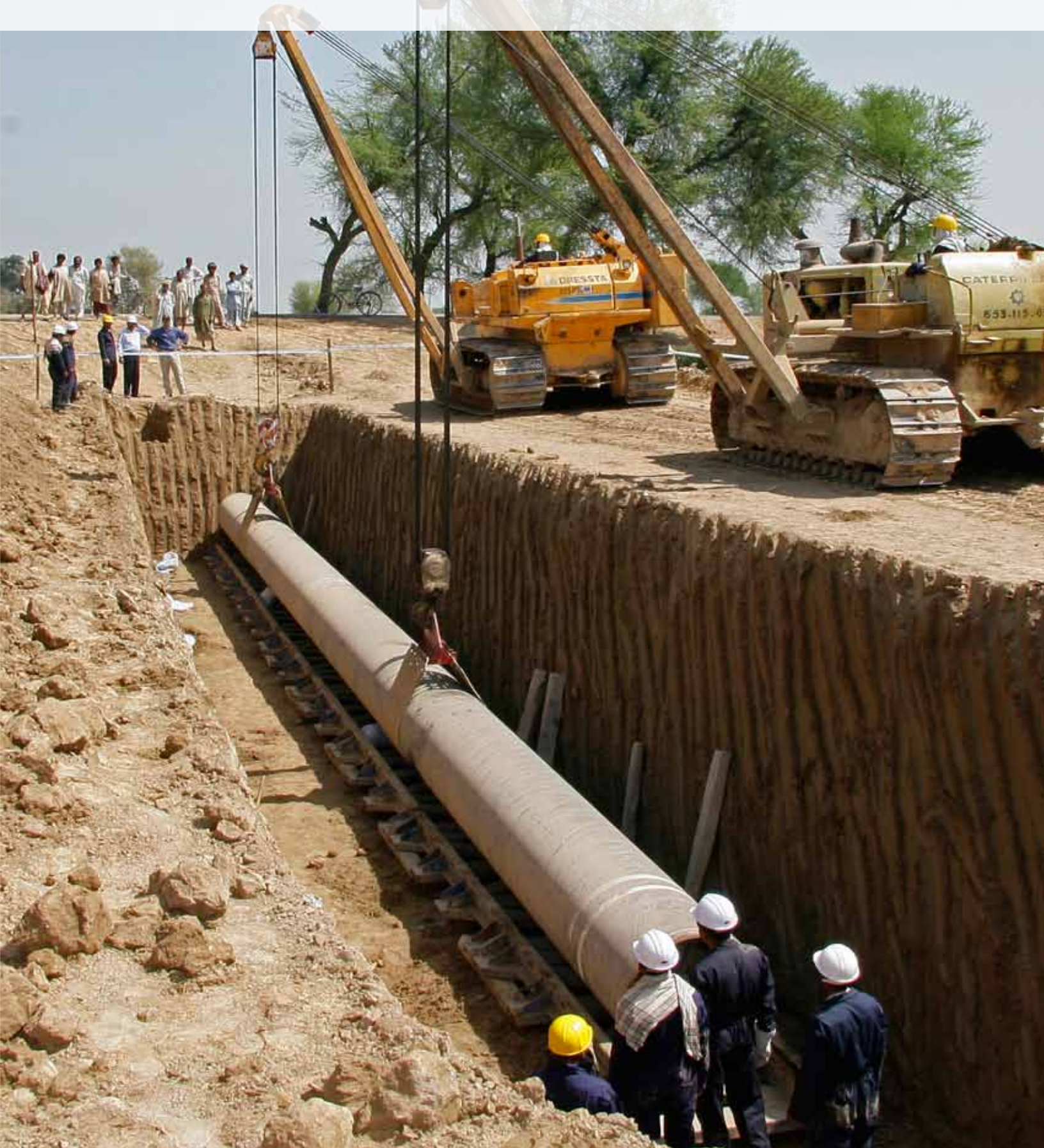
Preparation for thrust bore crossing (36" diameter gas pipeline Multan Road, Lahore).
