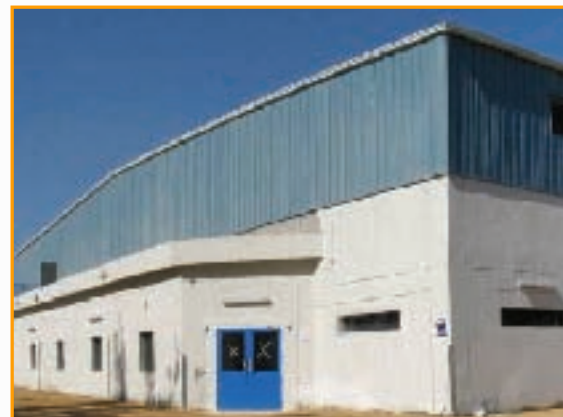
Liquids Transfer Project: external view of building
