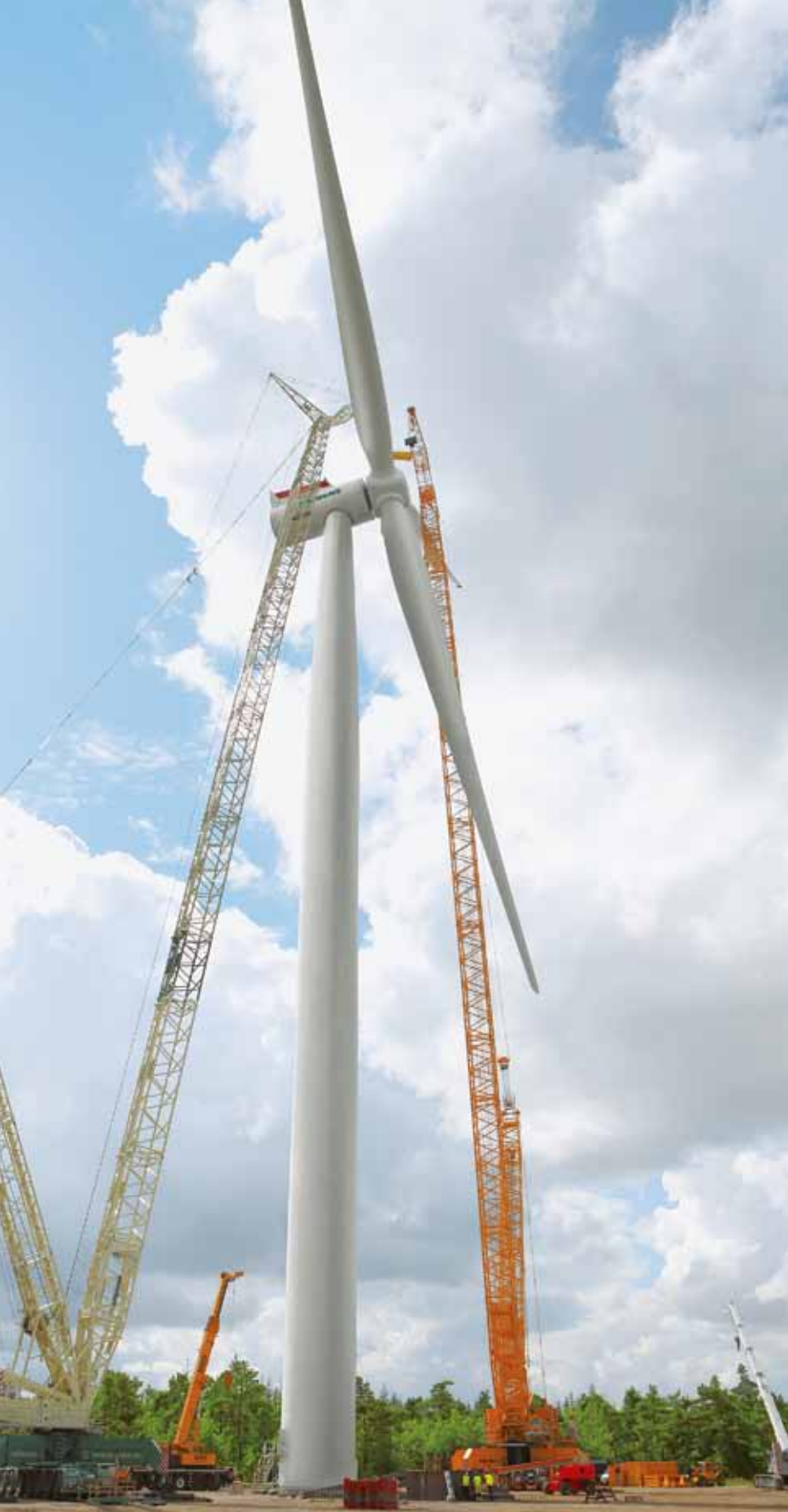
LEFT – A job well done: after two huge cranes have positioned the rotor – which has a total diameter of 154 meters – specialists connect it directly to the generator shaft.
