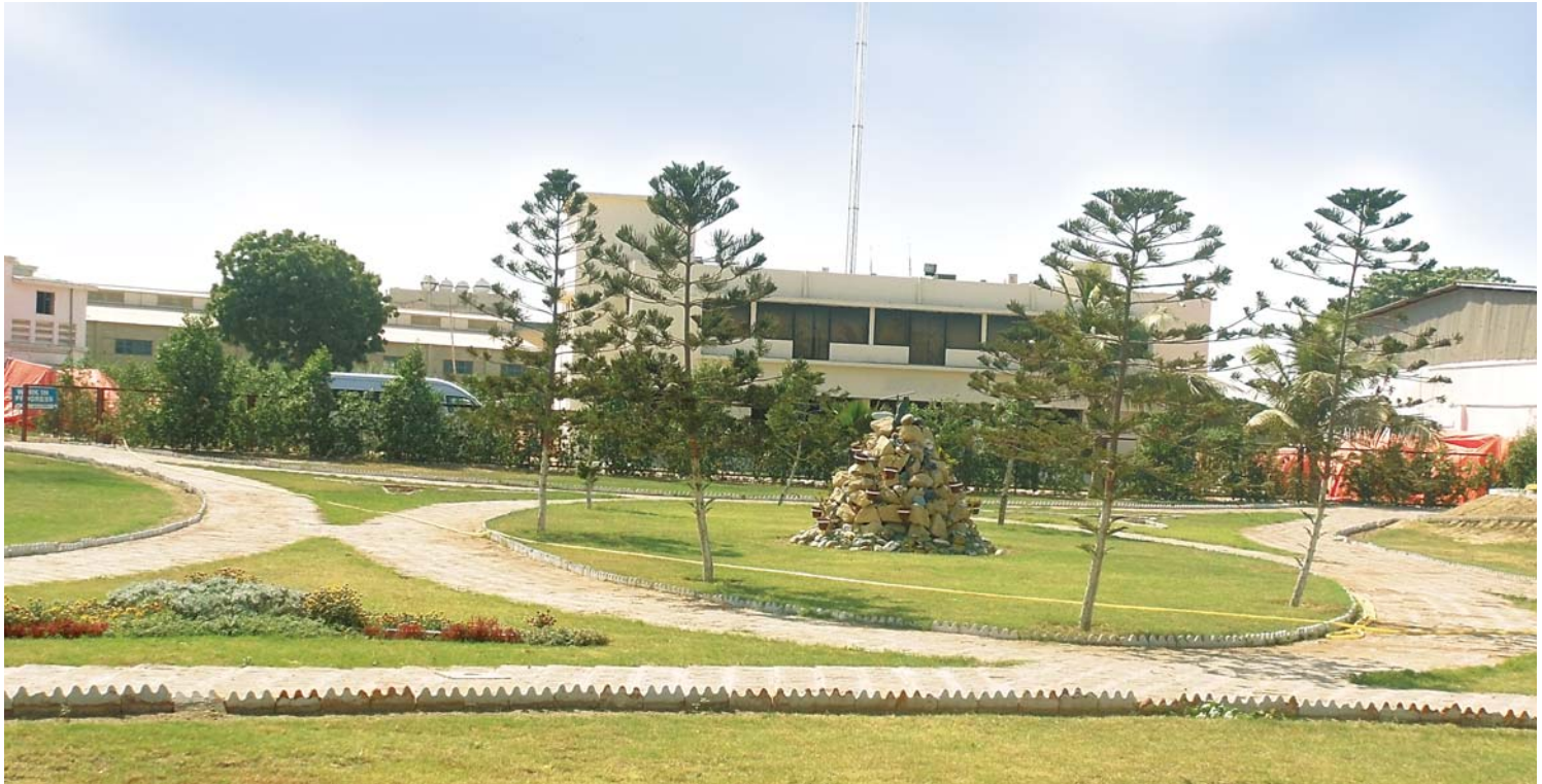
An inside view of AEL Factory
