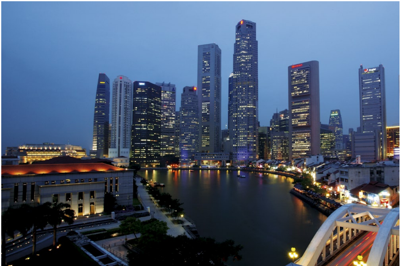
SP Group has transformed into a major utility infrastructure player in the Asia Pacific.
