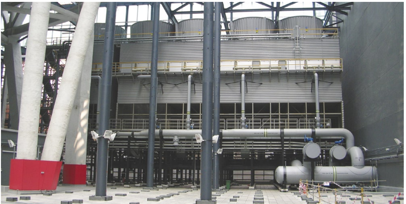
A centralised cooling tower eliminates the need for an in-house chiller plant in buildings.
