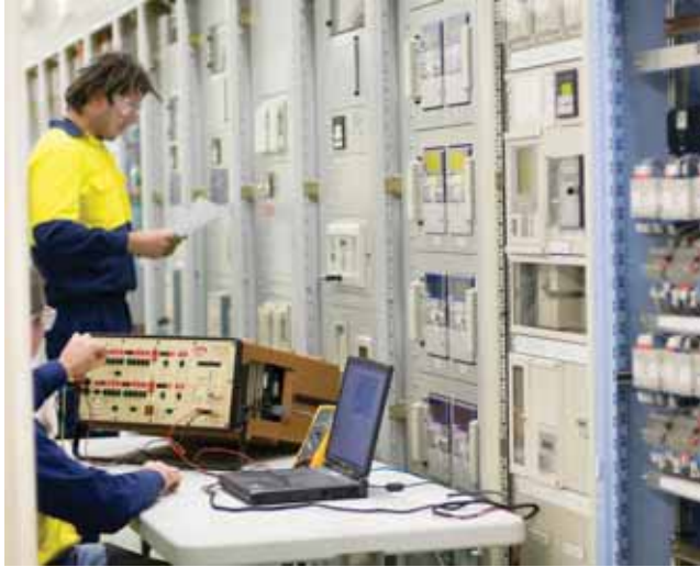
Working at the Altona Terminal Station
