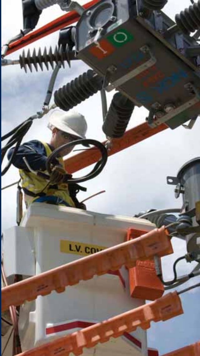
Electricity distribution line work underway in Lilydale
