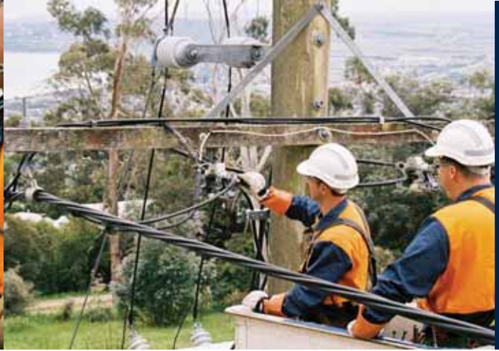
Fixing a powerline overlooking Port Phillip Bay, Mornington Peninsula
