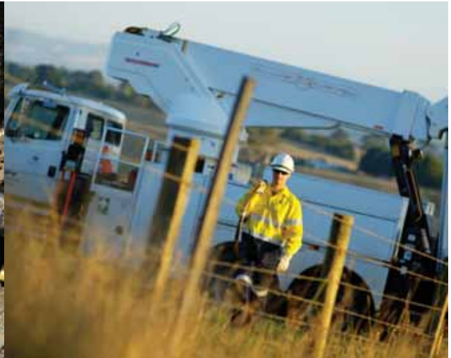
Warragul workers on an electricity distribution job
