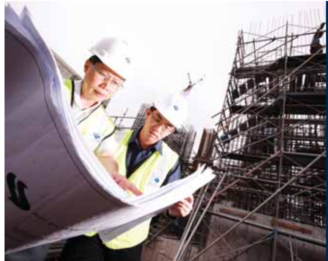
New substations being constructed to meet increasing load growth
