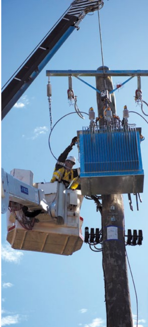
Fixing a power line in Melbourne.
