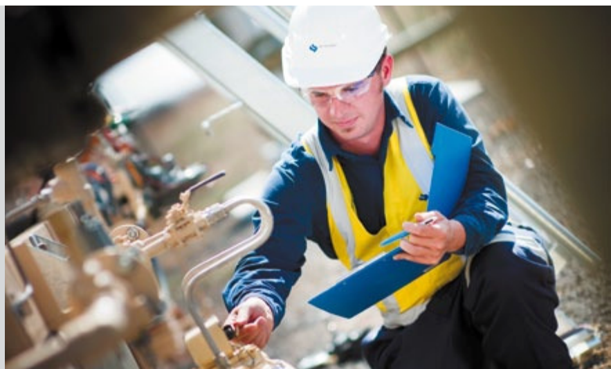
Gas distribution works with gas meters.
