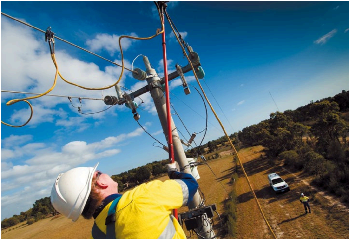
Undertaking maintenance works near Benalla.
