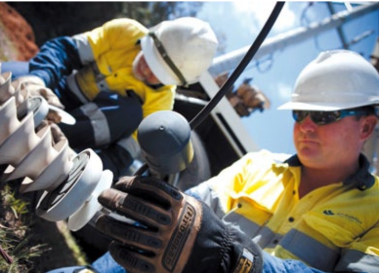
SP AusNet crew working on distribution insulators.
