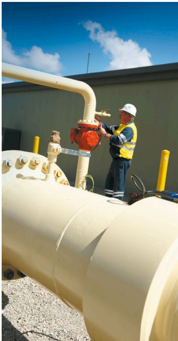
A Jemena worker conducts maintenance work on gas transmission pipelines.
