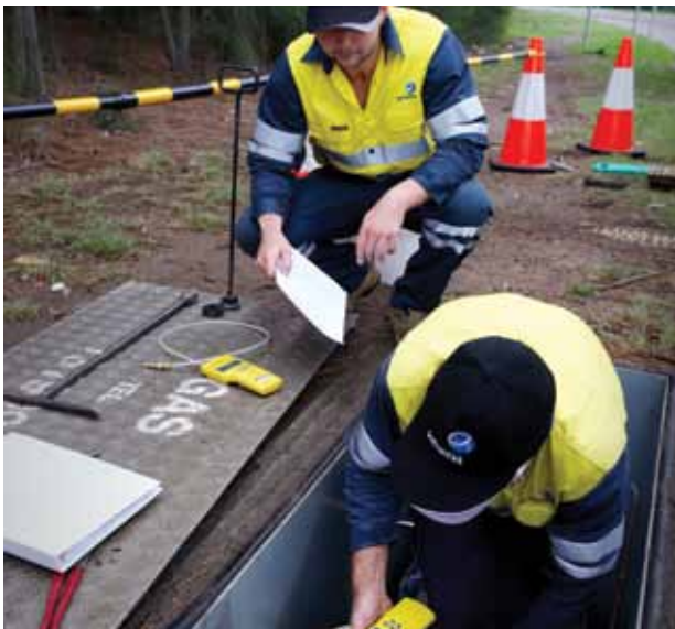
Technicians working on the Jemena Gas Network in Sydney.
