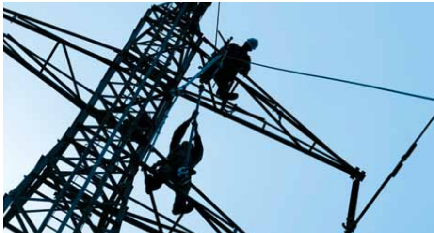
SP AusNet linesmen working on the electricity network.
