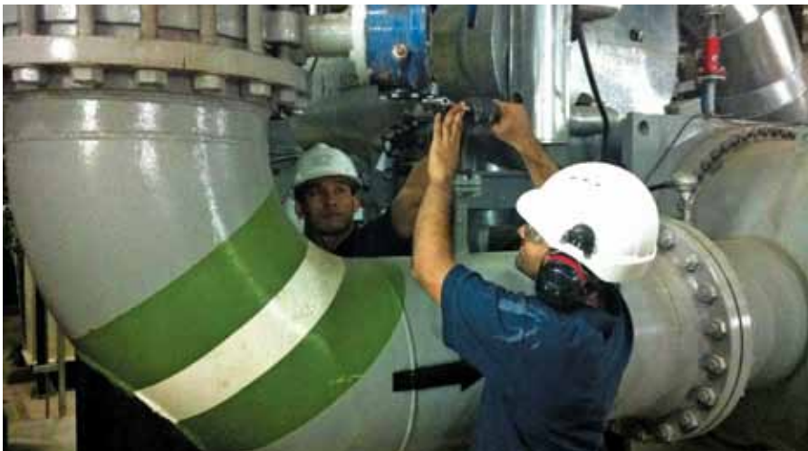
SDC technicians conducting maintenance of chiller systems.
