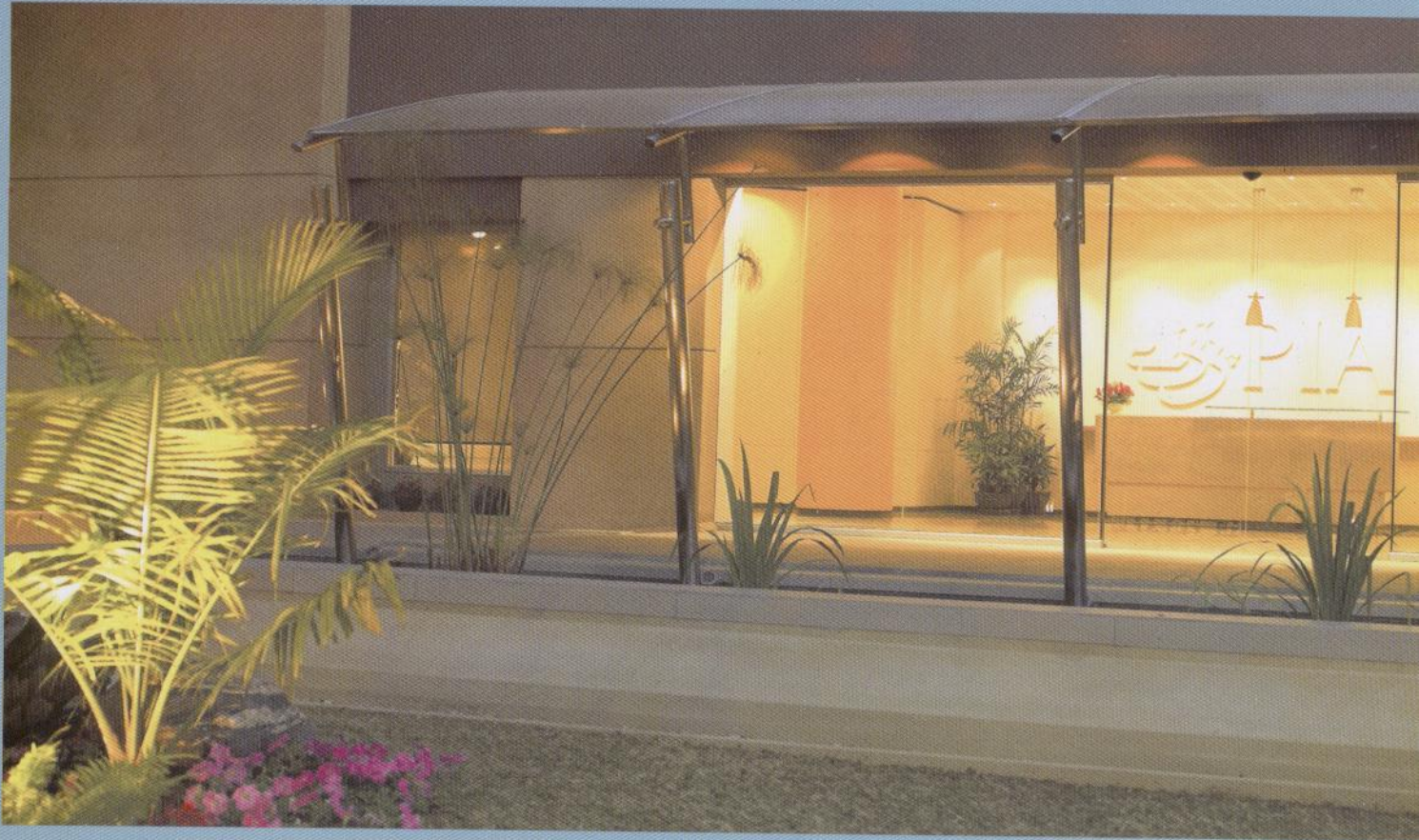
The new entrance of PIA's Corporate Office, Karachi.
