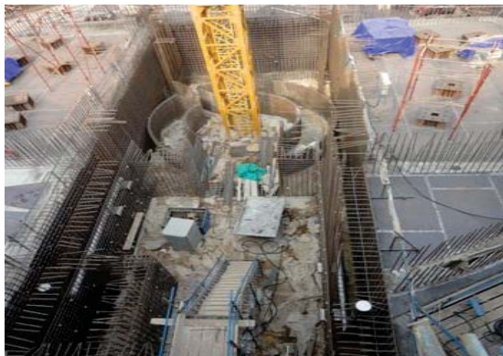
Inspection of Civil Construction Activities at C-3 Site
