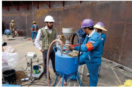
Inspections of Cement Grouting During Construction of C-3 NPP
