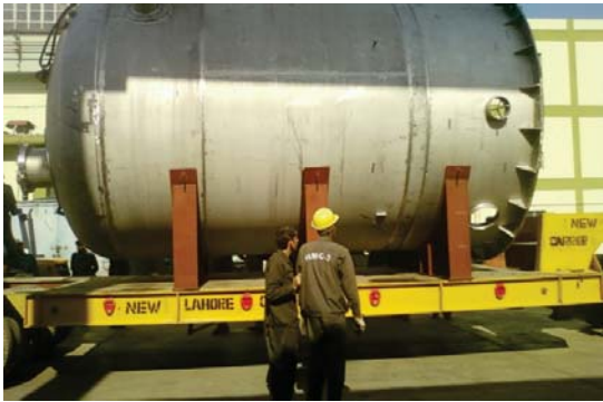
Inspection of Boric Acid Hold-up Tank
