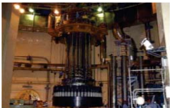
C-1 RPV Head Installation After RFO-7
