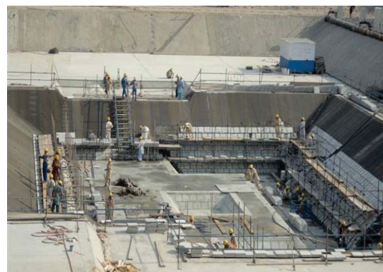
Nuclear Island Before First Concrete Pouring of C-4
