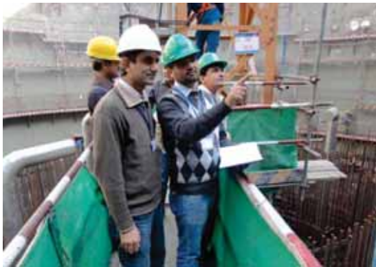
PNRA Inspectors at Under Construction Plant
