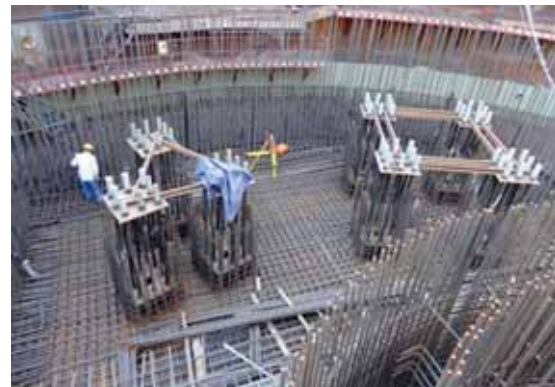
Steam Generator and Reactor Coolant Pump foundations
