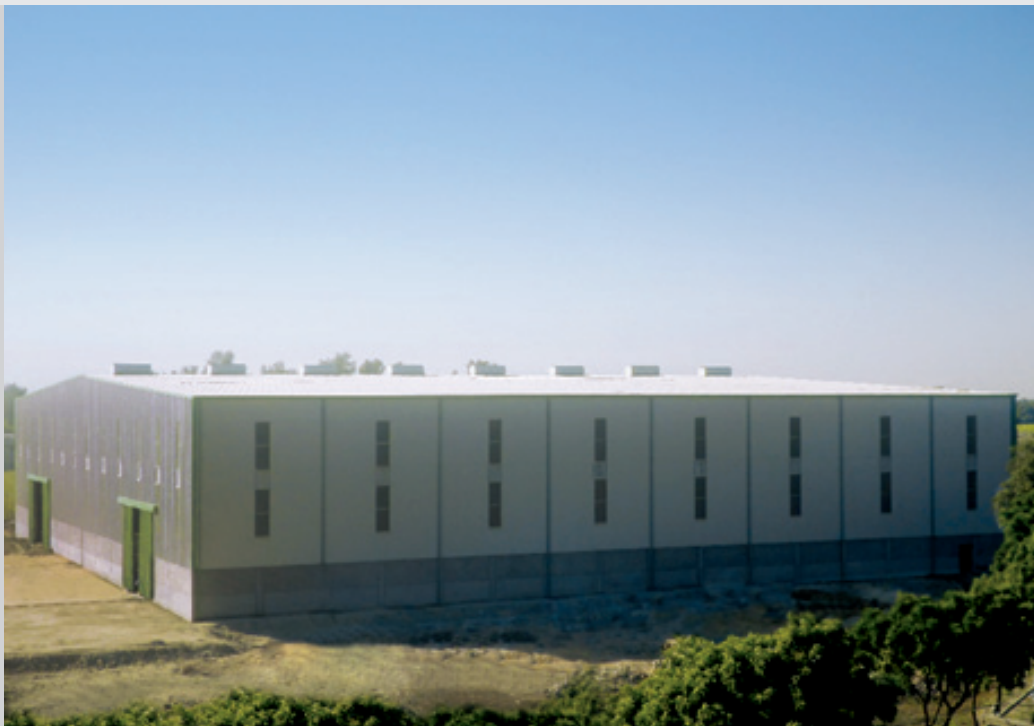
Our newly built 60,000 square feet Godown caters for 35,000 Tons of Sugar and shall be operational from crushing season 2013-2014.
