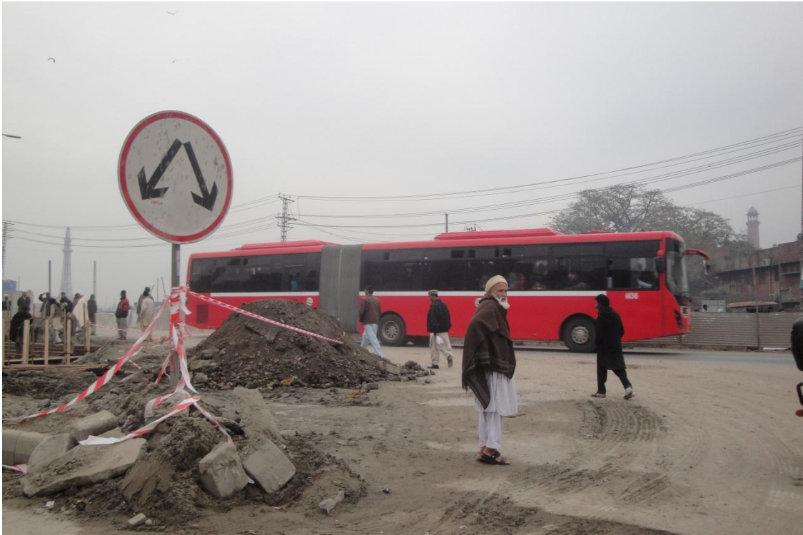
During Construction Phase of the Project
