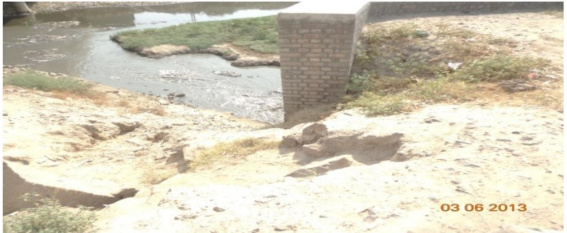
Fig.3.6: Tamery wastewater entrance in Pandoki drain.
