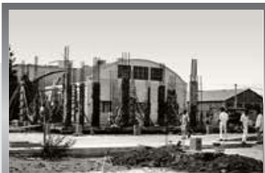
PCL factory being built.
