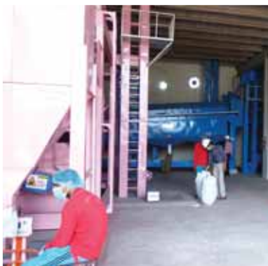
Recently commissioned Seeds Processing Plant
