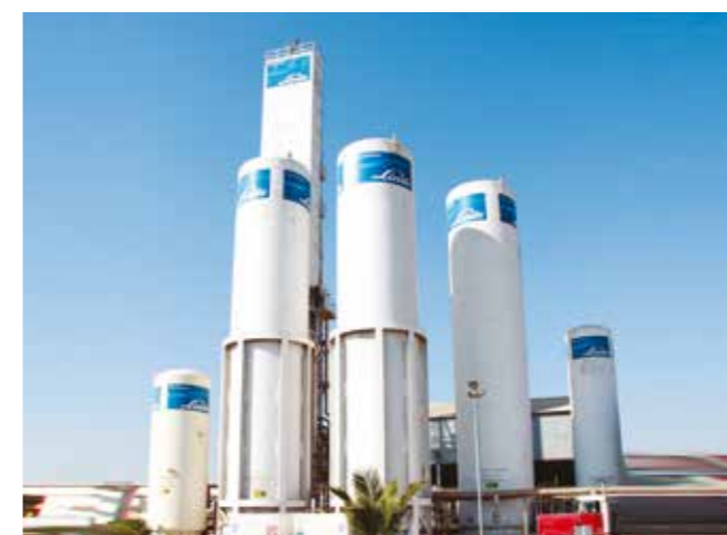
Successful relocation of ASPEN-1000 from Taxila to Port Qasim
