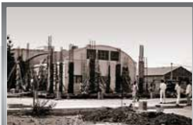
PCL factory being built.
