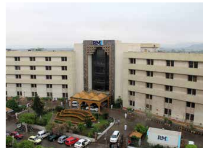
Linde successfully completed pipeline projects at major hospitals such as Rehman Medical Institute, Peshawar.
