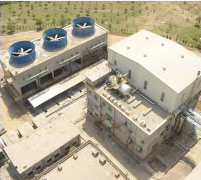
Waste Heat Recovery Power Plant
