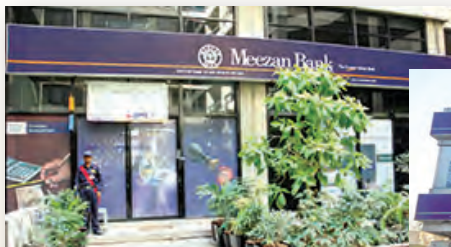
FTC Branch, Karachi - Meezan Bank's 1 st Branch
