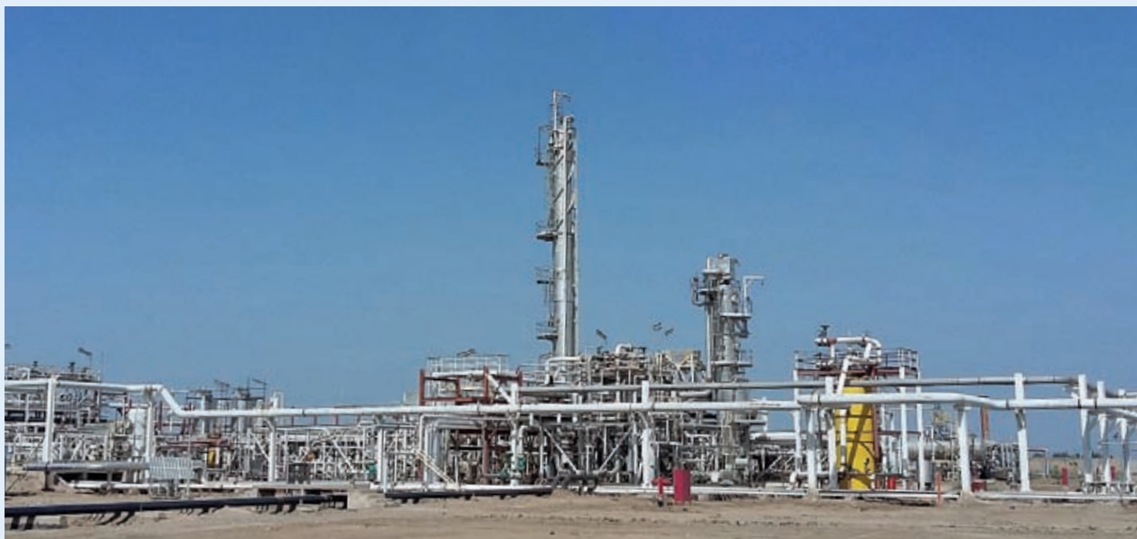
Sinjhero processing facilities, district Sanghar, Sindh.
