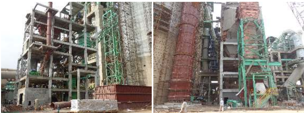
Rehabilitation Work in progress
