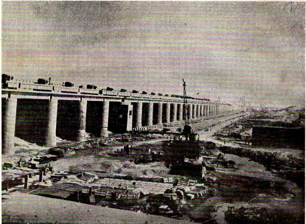
Guddu Barrage under construction
