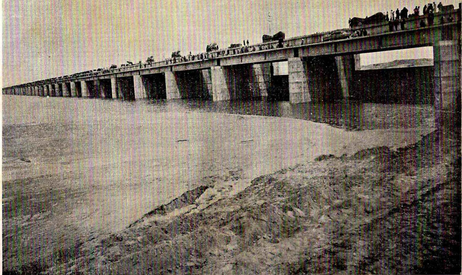
Guddu Barrage constructed by WAPDA. The Barrage will provide irrigation to 28,70,000 acres in the former Sind and Baluchistan areas. The Barrage has 1.2 million cusecs discharge and is 4,485 feet wide.
