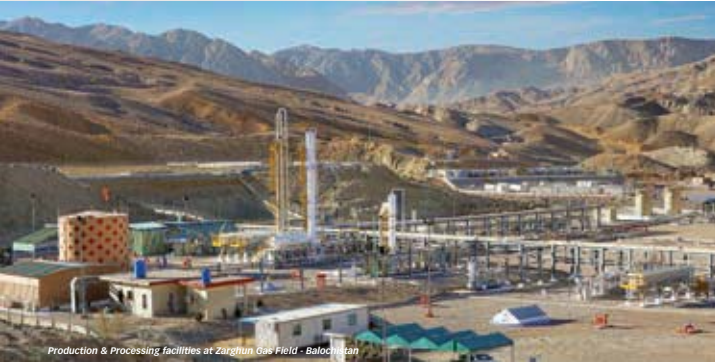
Production & Processing facilities at Zarghun Gas Field - Balochistan
