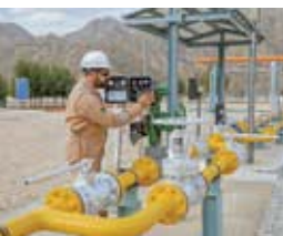
installation of compression package of 4 MMSCFD capacity.
