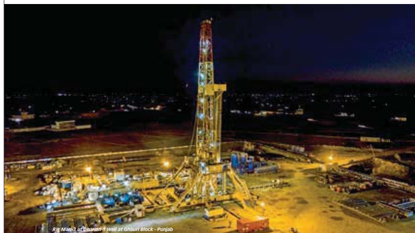
Rig Mari-3 at Dharian-1 Well at Ghauri Block - Punjab
