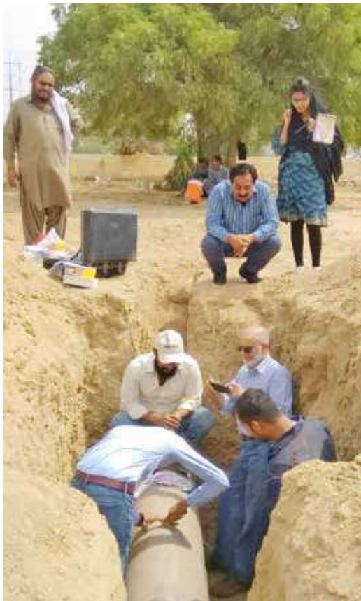
Inspection of applied Liquid Epoxy on 18" dia. IRBP Malir Cantt
