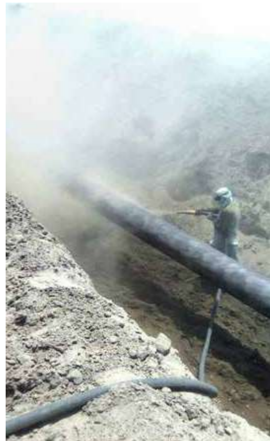
Sand Blast Cleaning of 16" dia. ILBP Shikarpur Section
