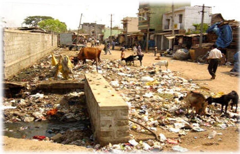
Figure 1-5: Animals scavenging organic material and clogged storm water drains
