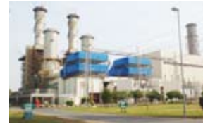
400 MW combines cycle power plant Block III at KAPCO
