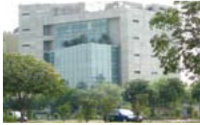
Electrical Health Check services to CDC House among other customers
