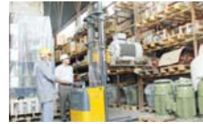
Motor store with the complete range of motors and alternators
