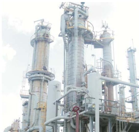
A view of plant to be relocated from Baton Rouge, USA. This will be the first ever EDC/VCM Plant in Pakistan
