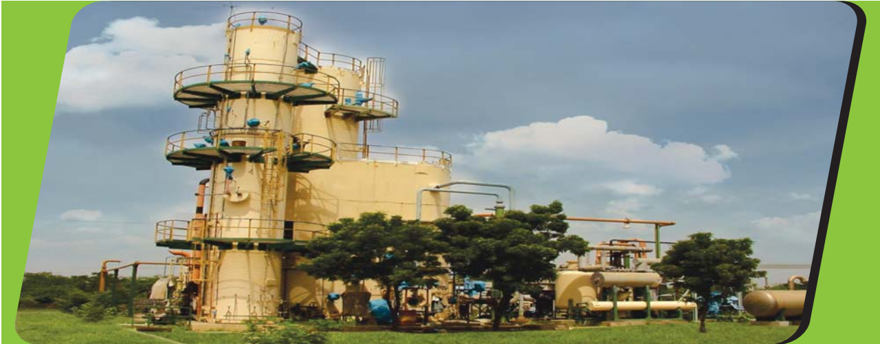
60 TPD PLANT VIEW
