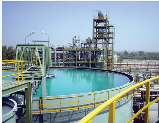
A view of new plant
