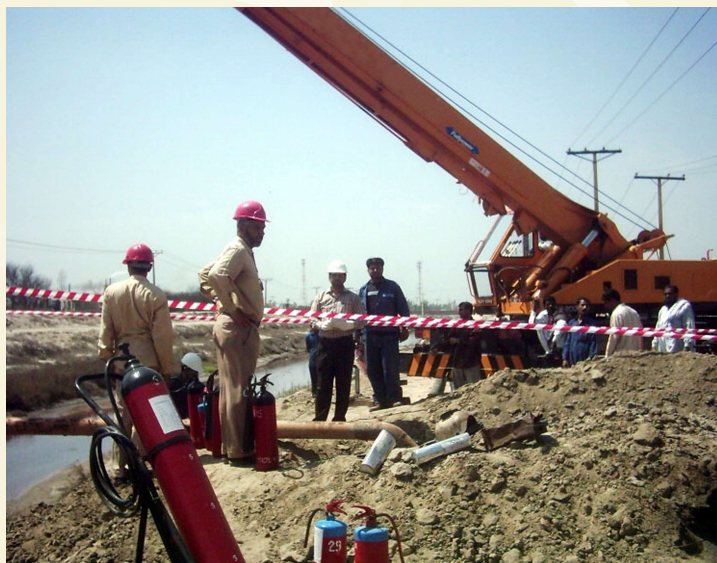
Work in progress for PVC plant construction
