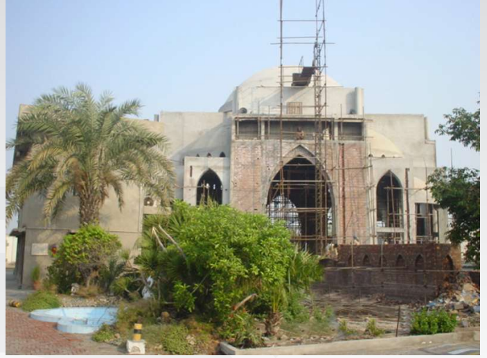
Under construction view of beautiful mosque at SCIL plant.
