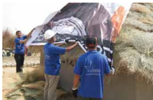
Our volunteers building a village in Thar
