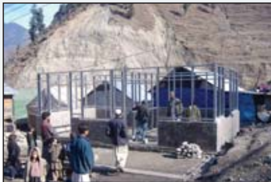
House under construction & ready for roofing
