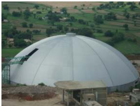
Raw Material Storage
