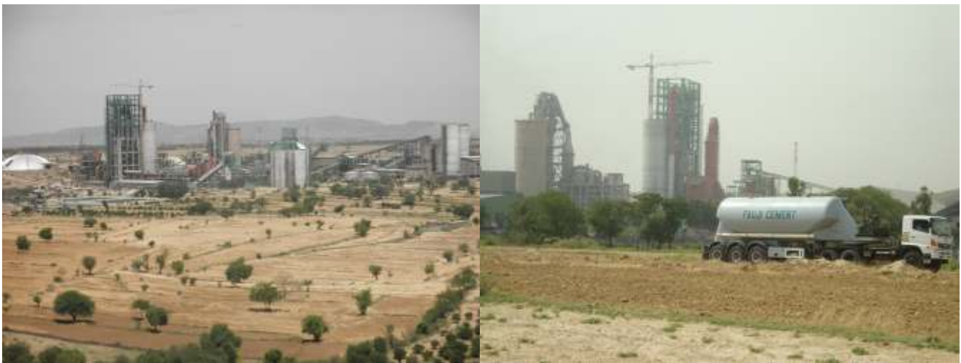
Overall Plant Picture.
