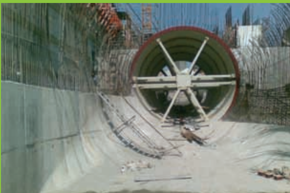
Laraib Plant - Tailrace Construction & Rotor Installation
