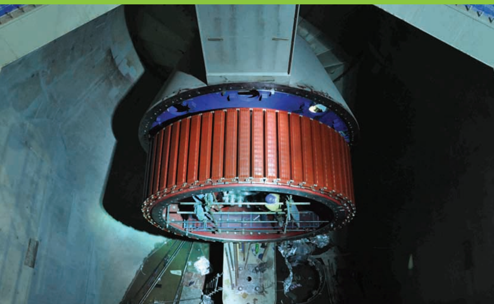
Laraib Plant - Installation of Generator
