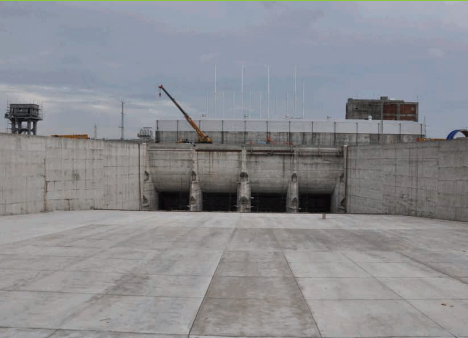
Laraib Plant - General View of Intake Slab
