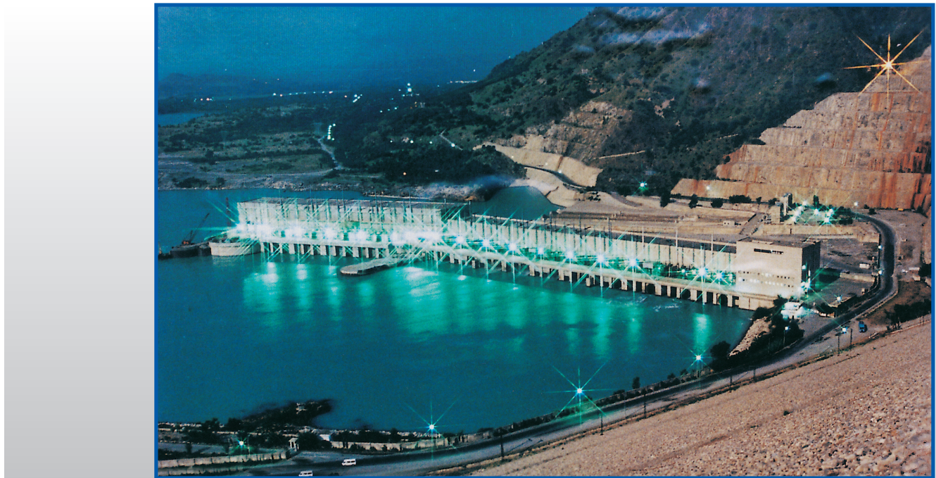
Tarbela Power House
