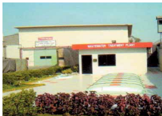
Waste Water Treatment Plant
