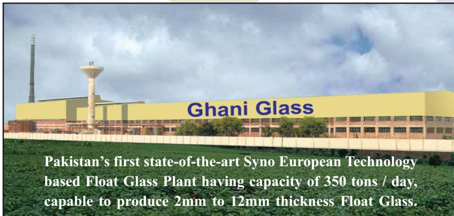
GGL-III SHEIKHUPURA (FLOAT GLASS MANUFACTURING PLANT)
