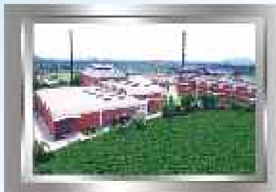
GGL-I HATTAR (CONTAINER GLASS MANUFACTURING PLANT)
