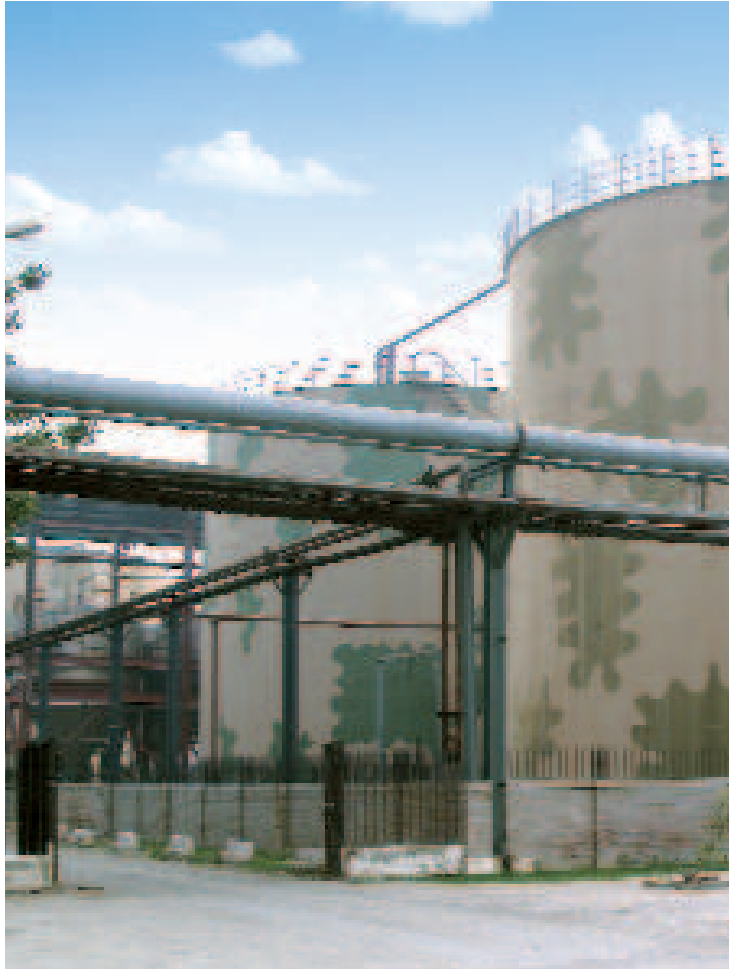
Molasses Storage Tanks along with steam water pipe lines used in ethanol manufacturing.
